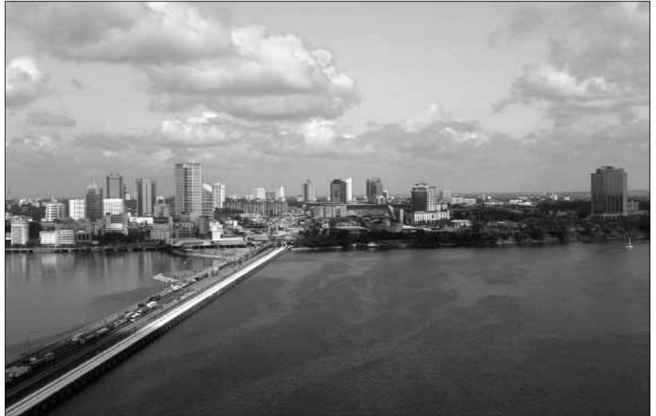
View of the embankment which connects Johor Bahru with Singapore. (picture Nicky Loh, reuters)
