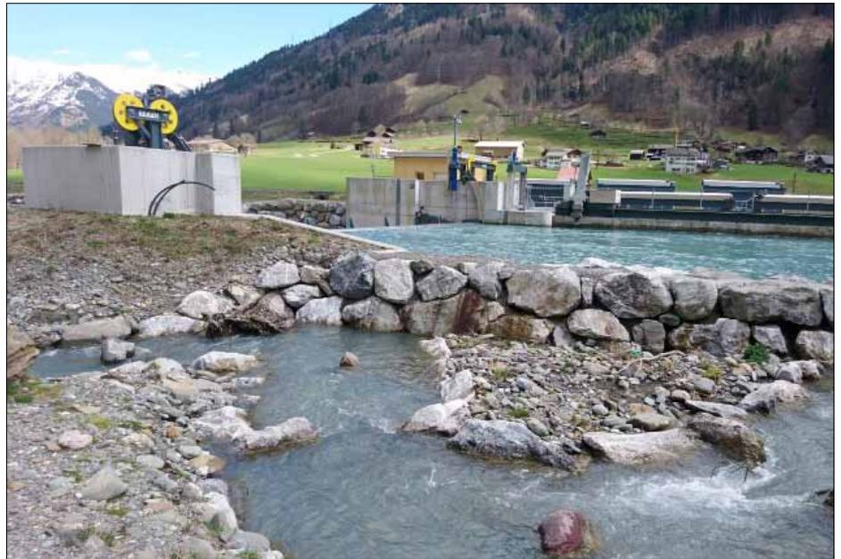
Rufi small power station (Glarus). In the foreground the bypass channel of the Rufi power station (GL) for the fish ladder. Behind it the weir and in the background the 3-chamber desander of the power plant. (Picture Swiss Small Hydro)
