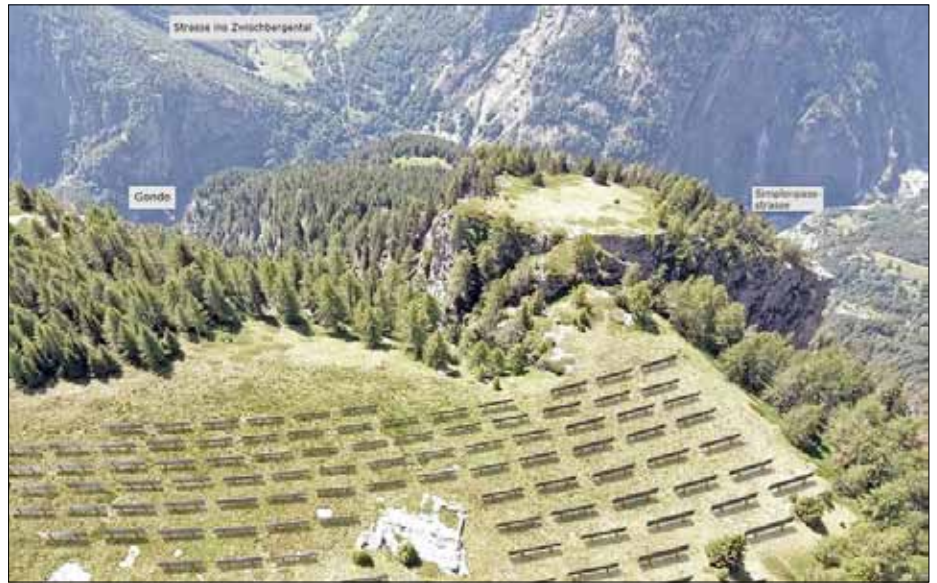
Solar System, Gondo in Wallis. (picture gondosolar)
