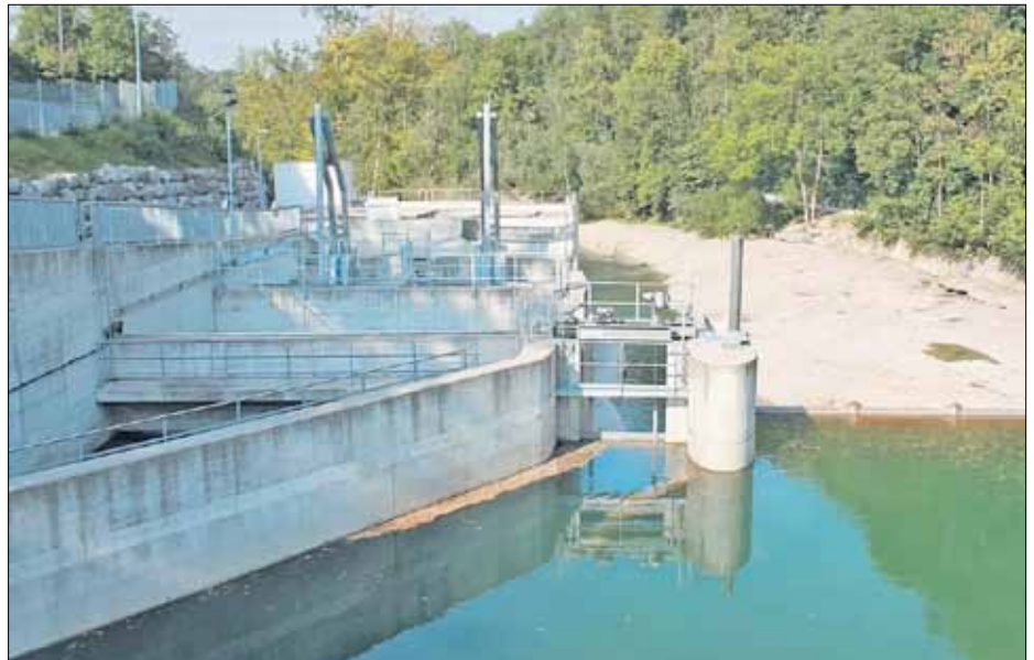
River power plant on the Thur in Bazenhaid in the canton of St. Gallen. (picture rwt)
