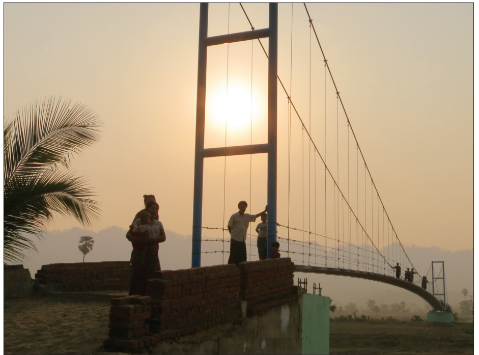
The bridges unite people with each other and are indispensable for coping with everyday life. They make adequate medical care possible, and the safe route to school opens up access to education for children. (picture Toni Rüttimann)
