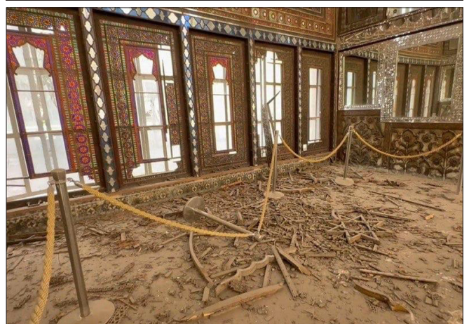
The Golestan Palace in Tehran, a UNESCO World Heritage Site: exterior view and the Throne Hall before and after a US-Israeli missile strike. (pictures Press TV)
