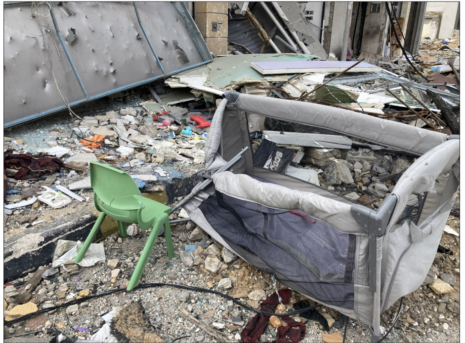
A shop selling baby products, completely destroyed following an Israeli air strike in southern Beirut. In the foreground, a destroyed cot. (picture Karin Leukefeld)
